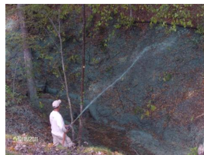
Ravine 3 - During Restoration
