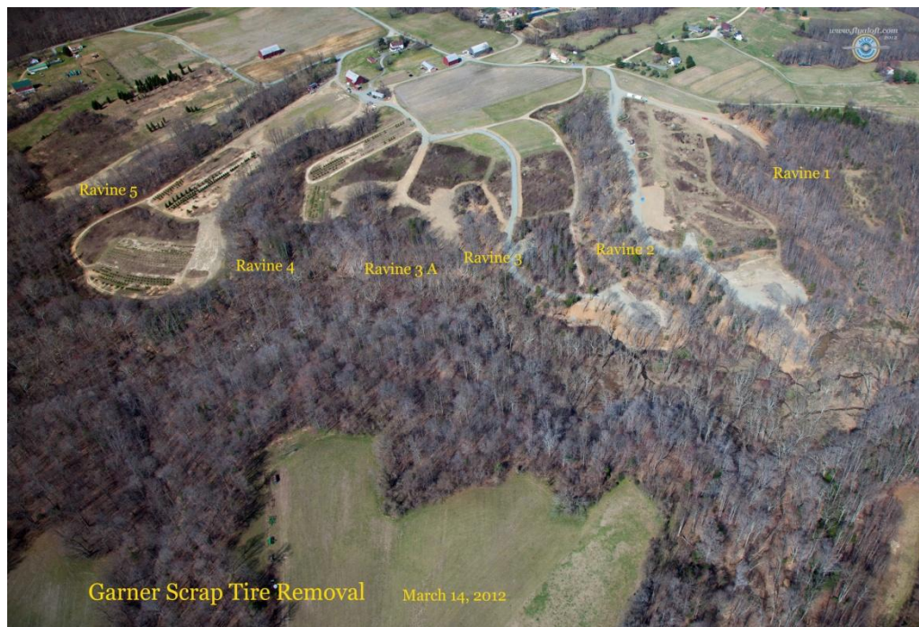
Aerial Photo of Entire Site During Cleanup
