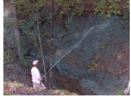
Ravine 3 - During Restoration
