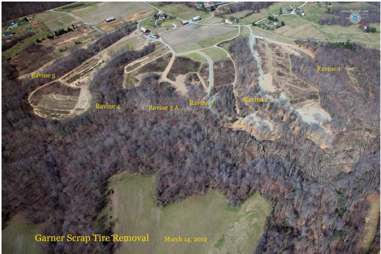
Aerial Photo of Entire Site During Cleanup
