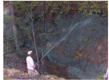
Ravine 3 - During Restoration
