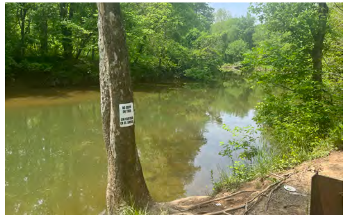
Signage and creek bank destabilization.
