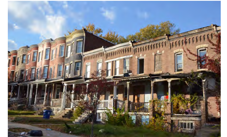
Figure 20 Porchfront-style rowhomes along West North Avenue.
