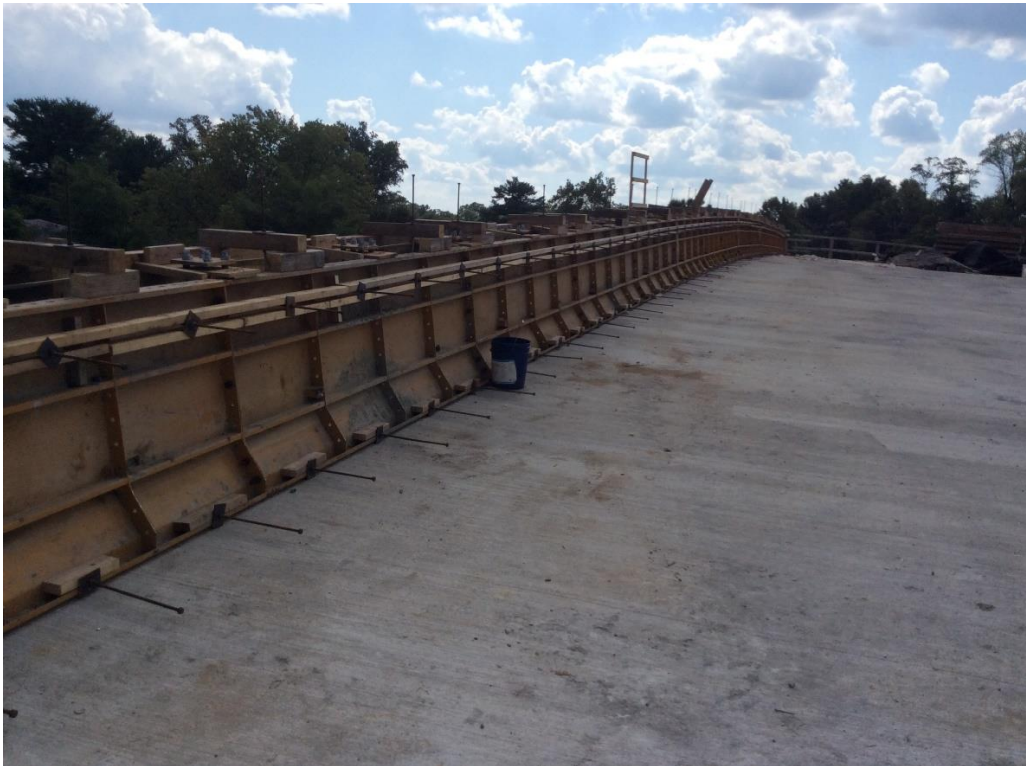
Segment 3 – Structure S20 LRT Bridge Deck Span 4 Concrete Placement at Silver Spring Transit Center (09/22/23)
