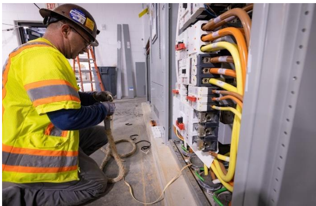
MC Dean and Pepco crewmembers adjusting cable inside the Glenridge Operations and Maintenance Facility in preparation for the move to full-power. The facility will serve as the hub of the Purple Line.
