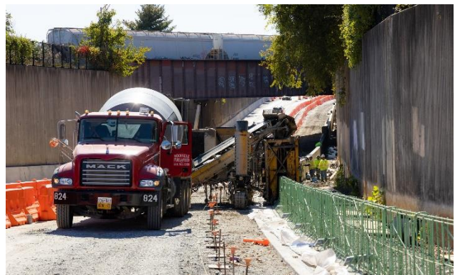
Construction of a barrier wall on Campus Drive at the University of Maryland, College Park to provide separation and protection for pedestrians using the sidewalk along the south side of the Campus Drive underpass.
