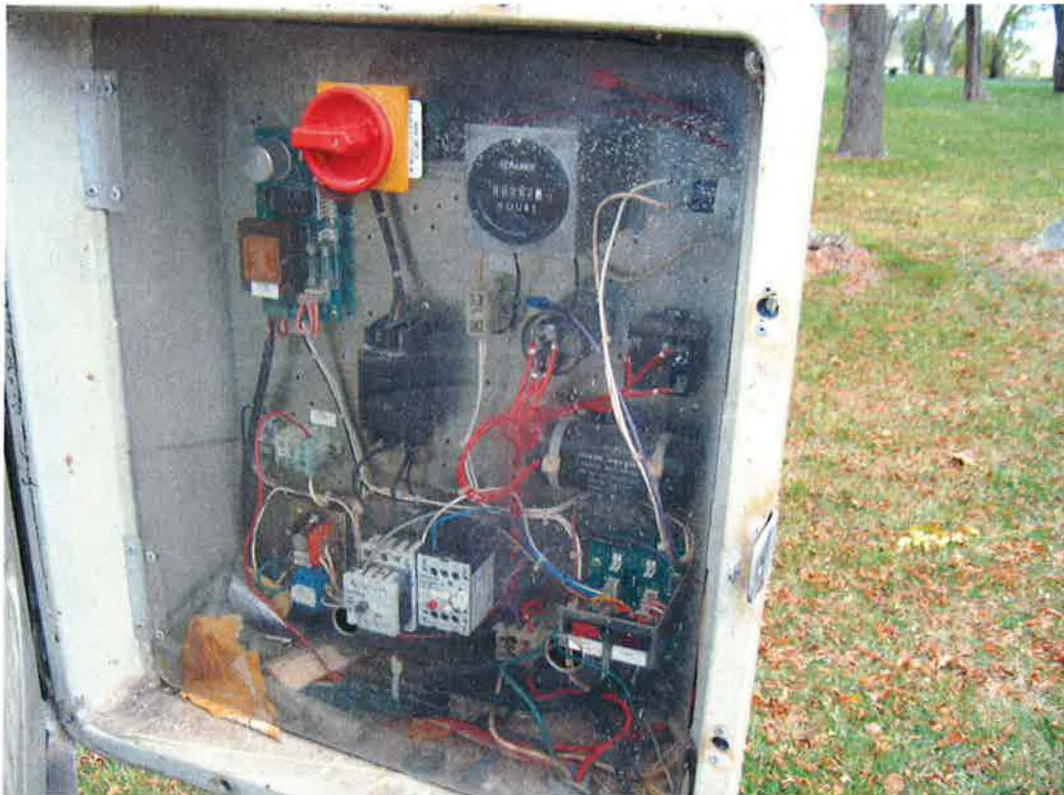
Grinder Pump Station Control Panel
