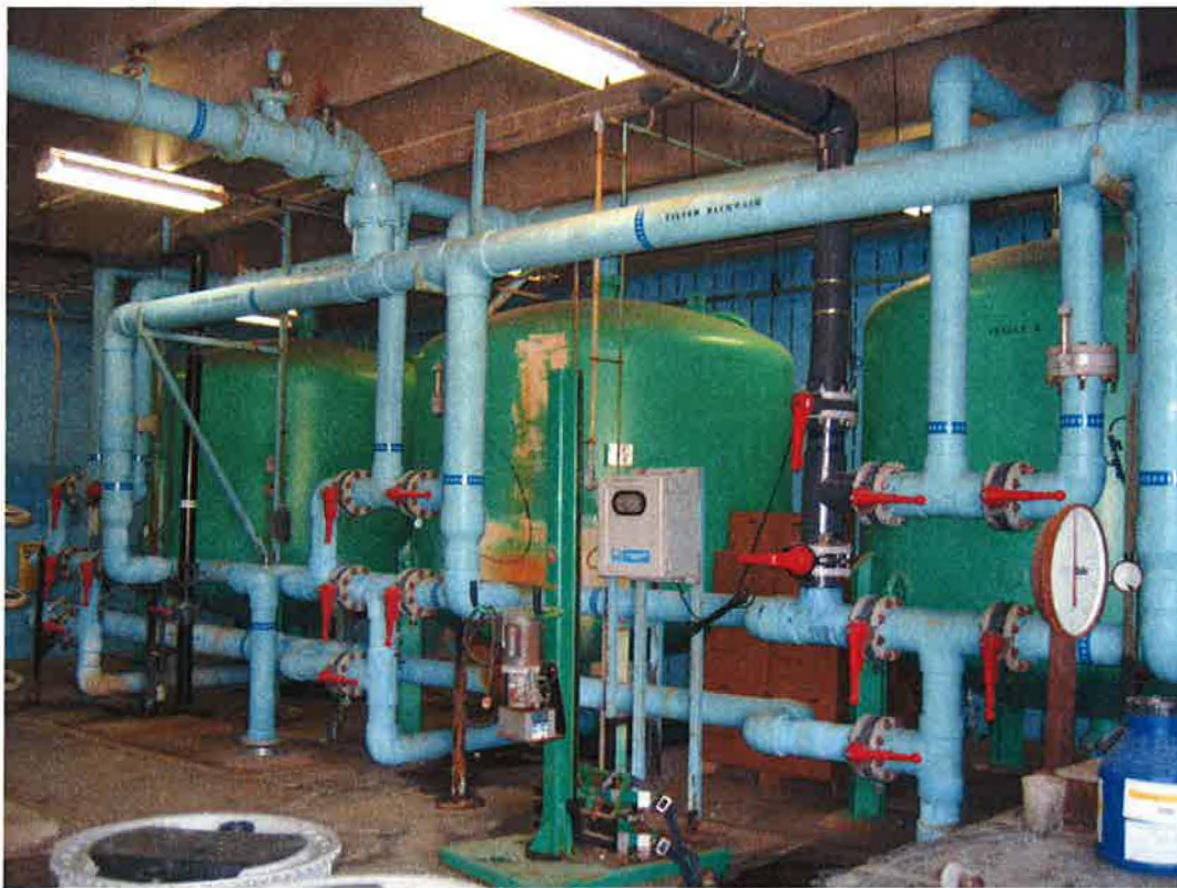
ECI WTP Greensand Filters
