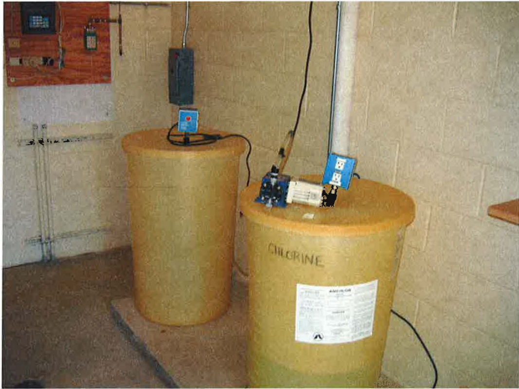
Sodium Hypochlorite Feed System
