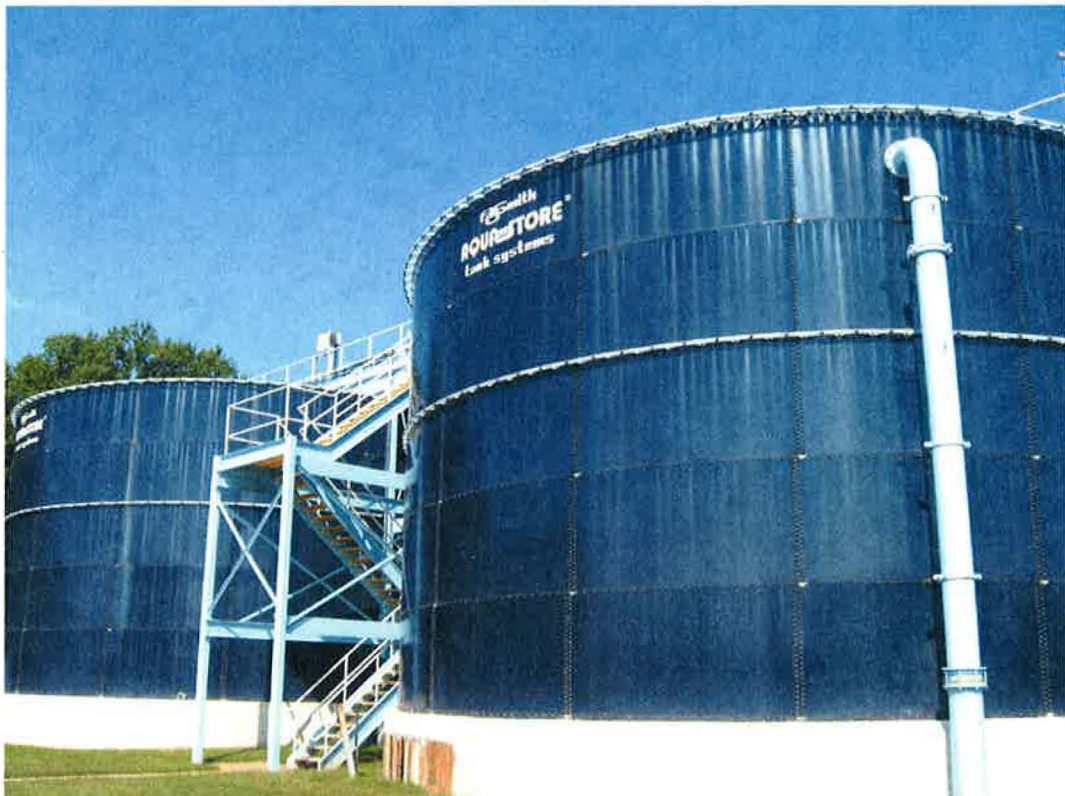
Flow Equalization Tanks
