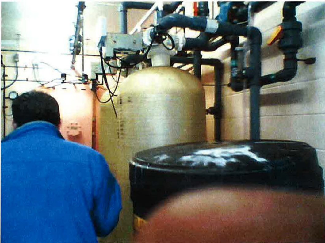
Ion Exchange Units
