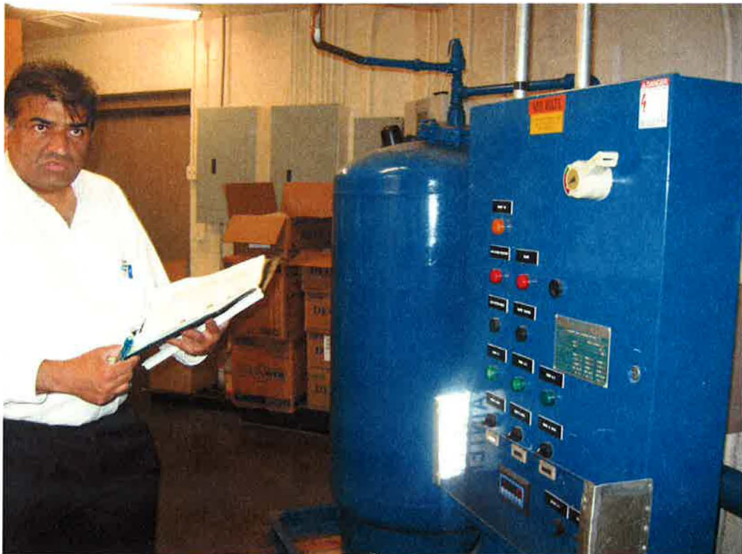
Bladder Tank and Controls- Eastbound
