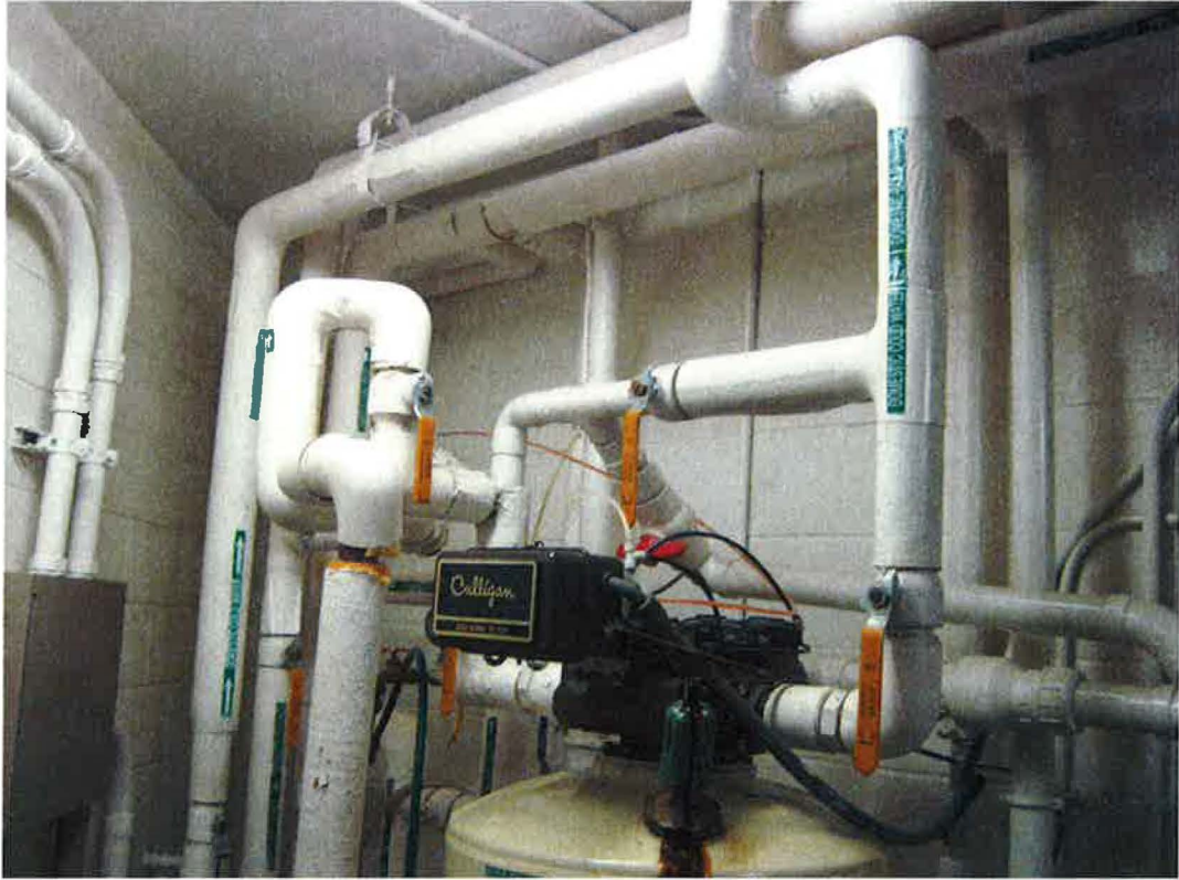
Greensand Filters and Process Piping-Eastbound
