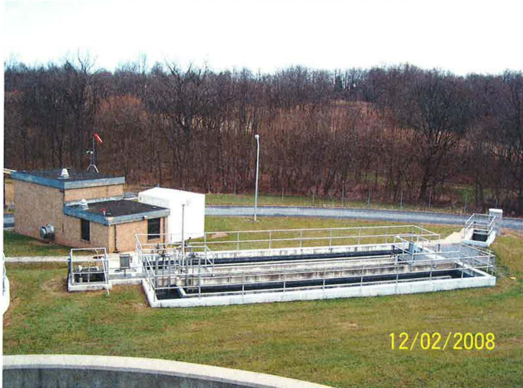
Chlorine and Sulfur Dioxide Treatment Units
