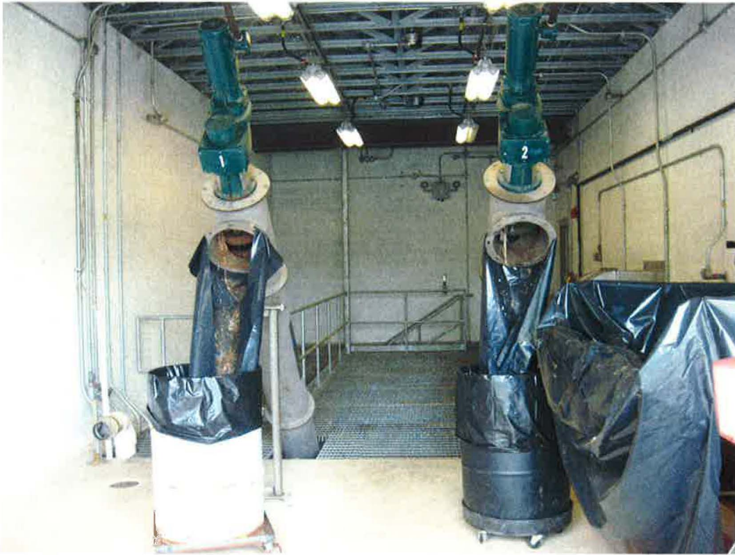
NBCI Screening Screw Compactor
