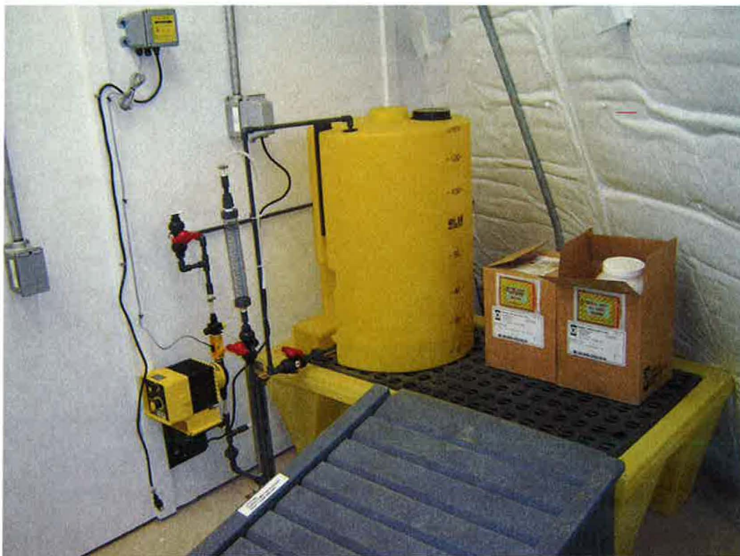
Sodium Hypochlorite Feed at Well Number 6
