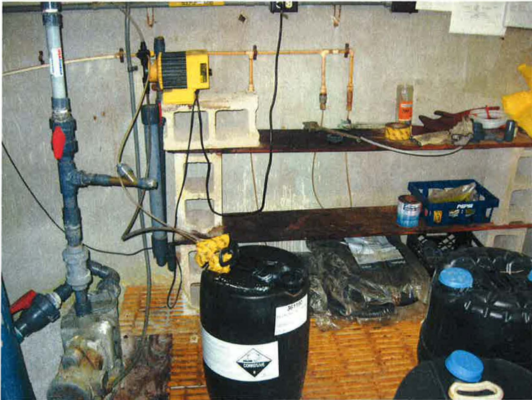
Sulfuric Acid Feed System
