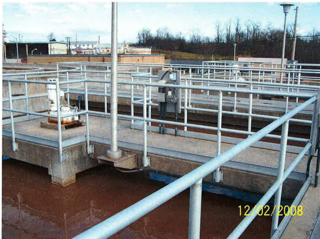
BNR Secondary Anoxic Tank
