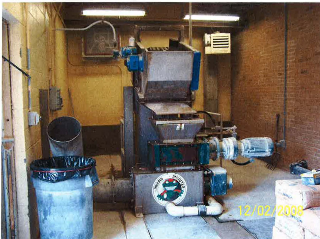
Headworks Muffin Monster and Bar Screen
