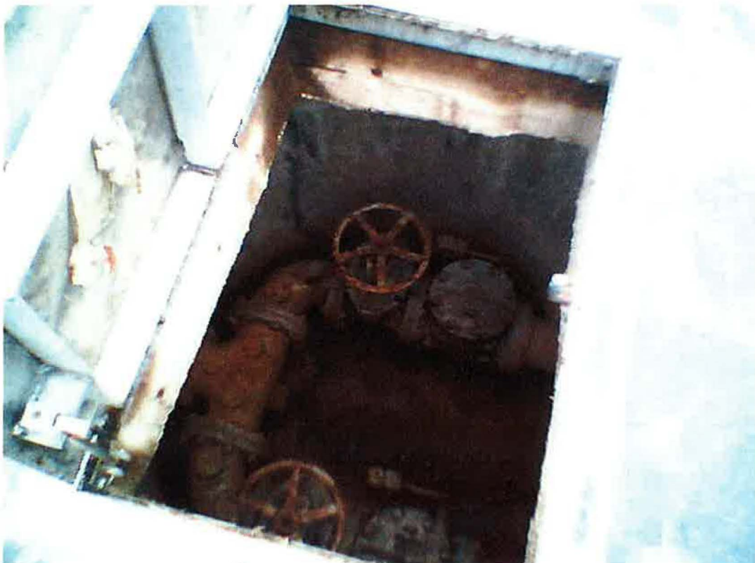
Sewage Pump Station Valves
