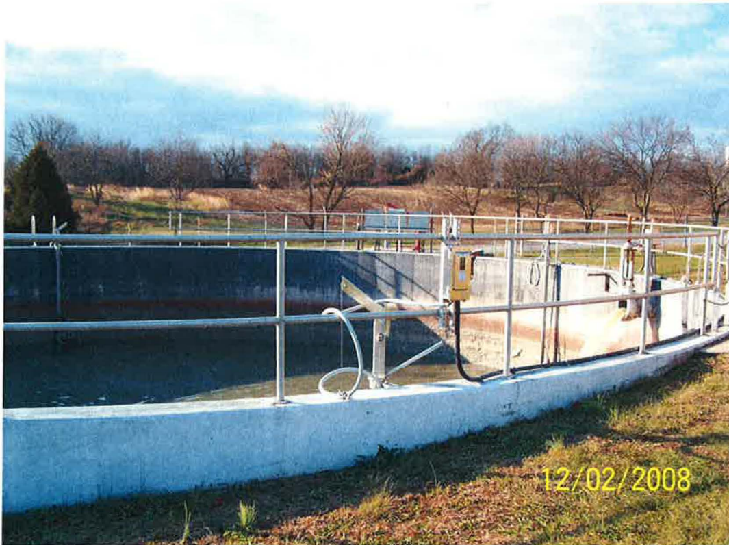
Flow Equalization Tank
