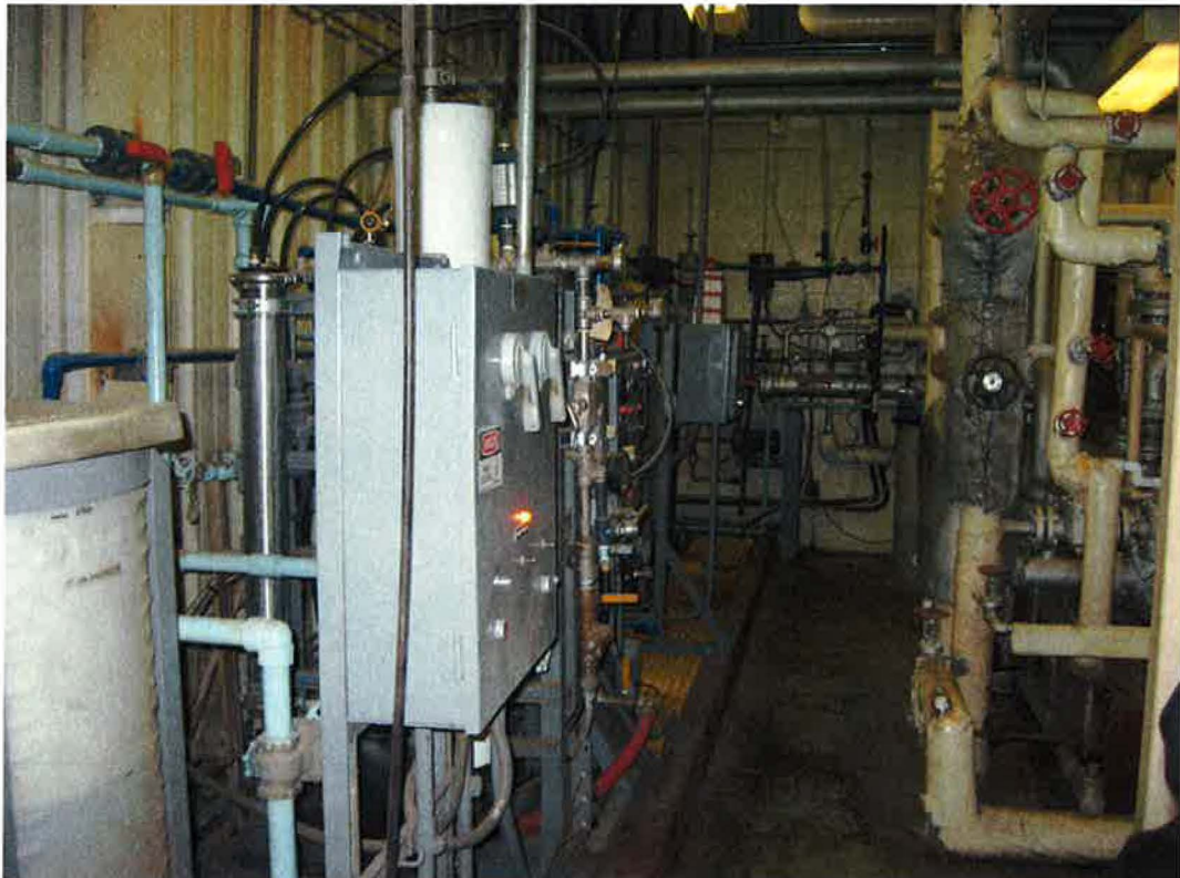
Boiler Make Up Water System
