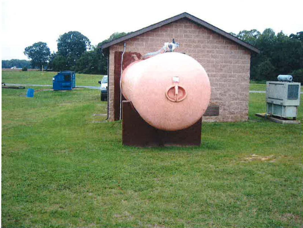
5,000-Gallon Hydropneumatic Tank
