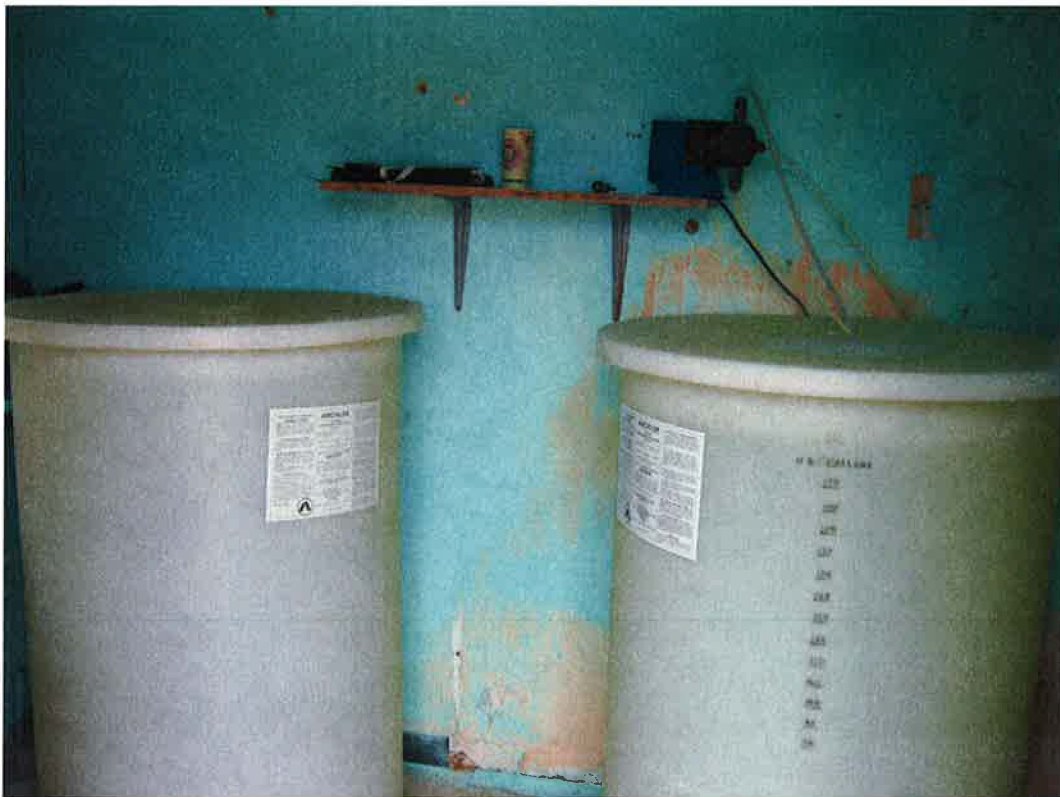
Sodium Hypochlorite Feed System
