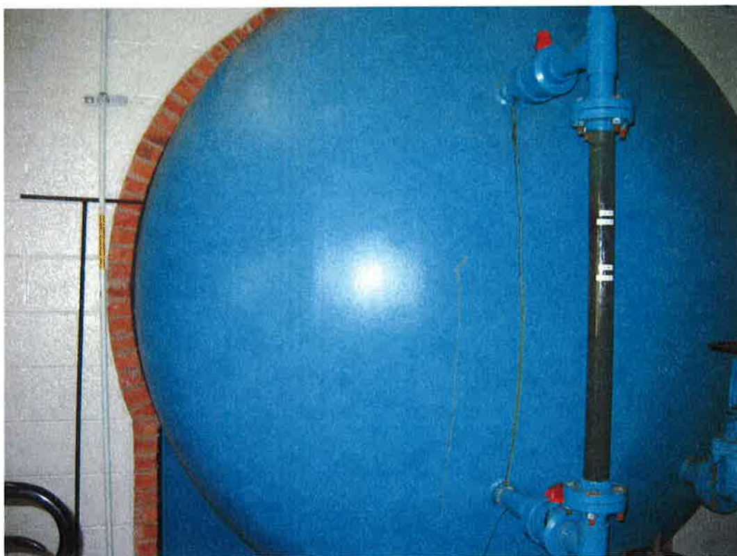
Hydropneumatic Tank
