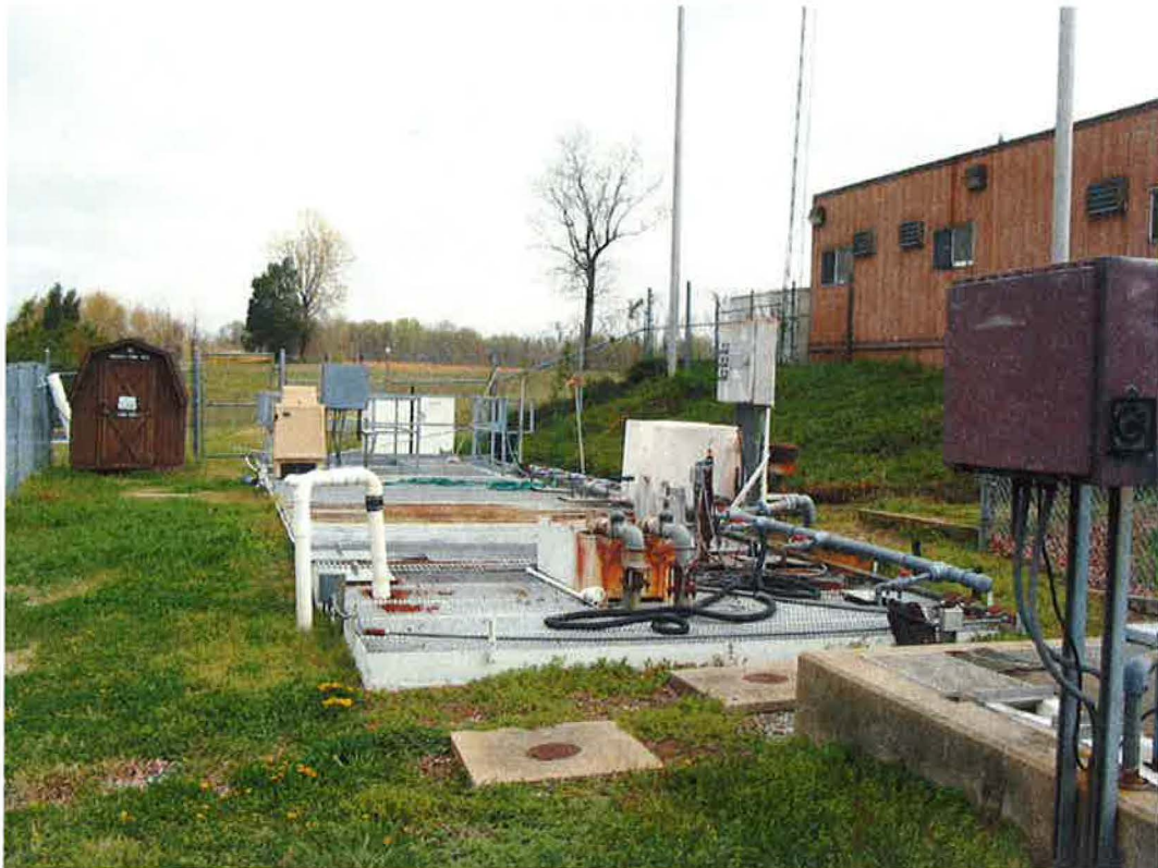
Wastewater Treatment Piping Corrosion
