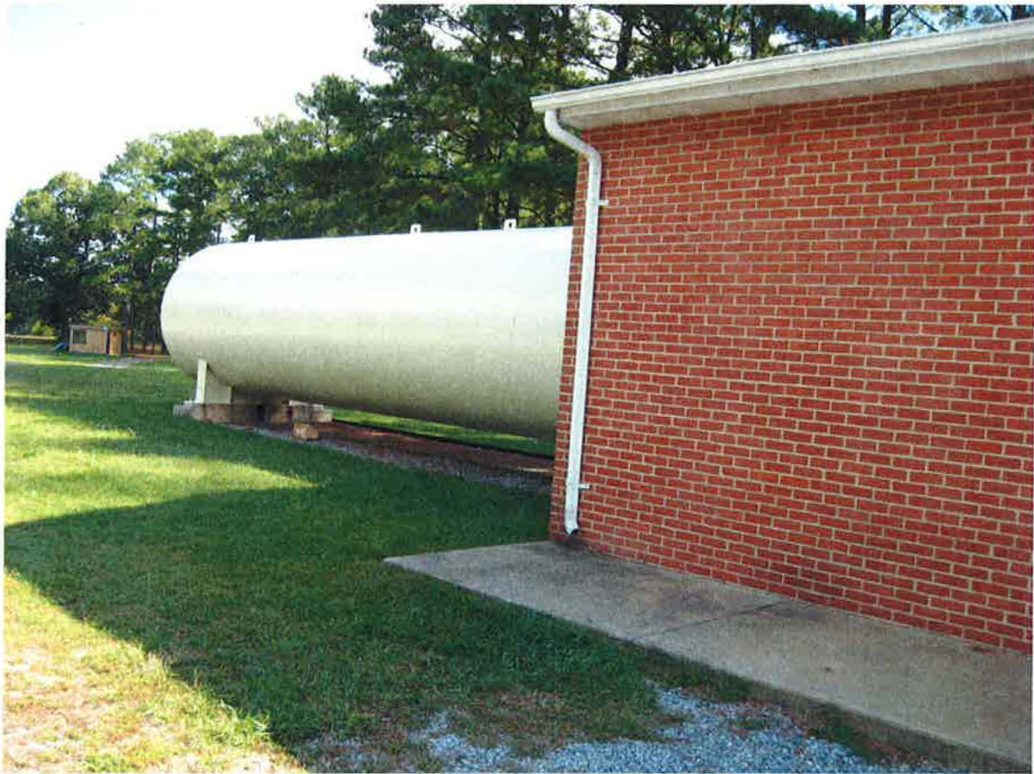
15,000-gallon Hydropneumatic Tank
