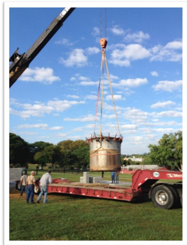
A vat from the Carroll County Farm Museum’s wormseed oil distillery being lowered onto a truck to make way for reconstructing the distillery’s pavilion. Photo courtesy of Carroll County Farm Museum.
