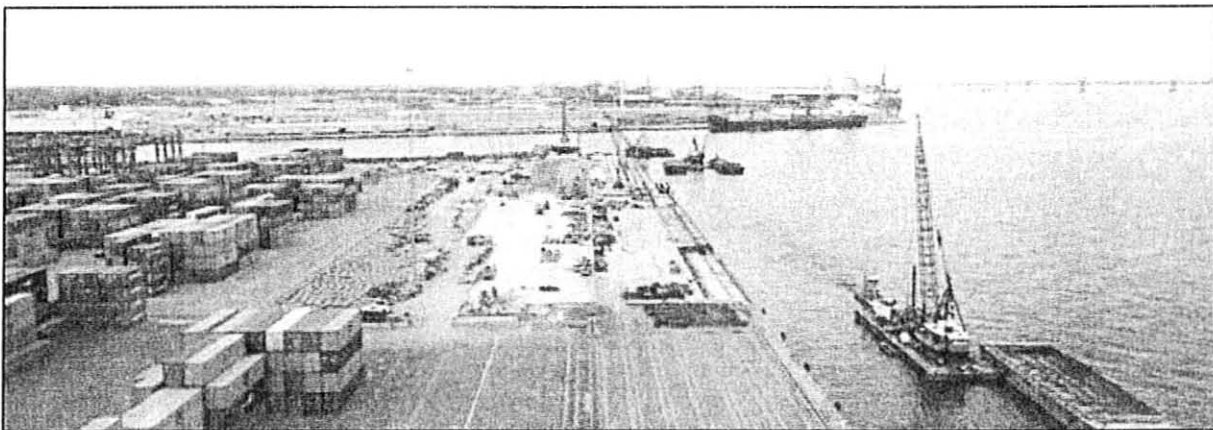
Construction progresses at Seagirt Marine Terminal Berth IV.
