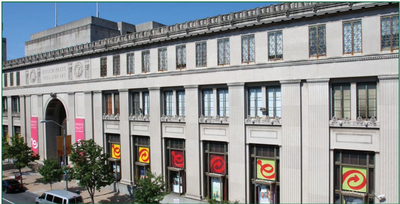
Enoch Pratt Free Library Central Branch Renovation, Baltimore, Maryland
