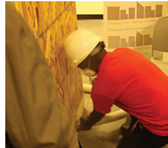
Weatherization demonstration - baltimore, 2010
